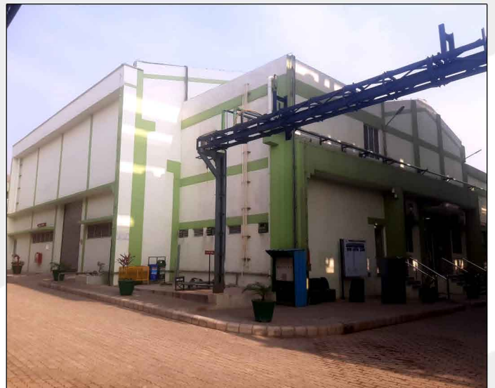
Compressor House Outside
