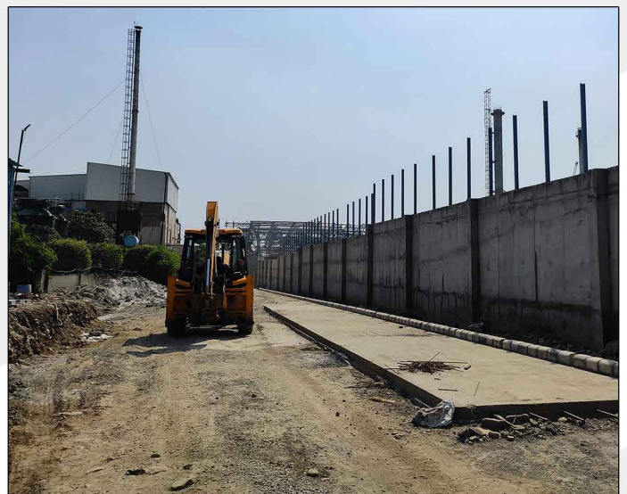
Husk Shed Open Area Boundry (40 TPH Boiler)
