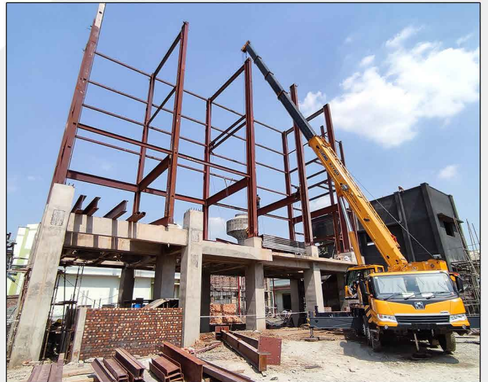
M.E. Building (R.O. PLANT)
