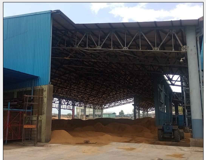
40 TPH Boiler Husk Shed
