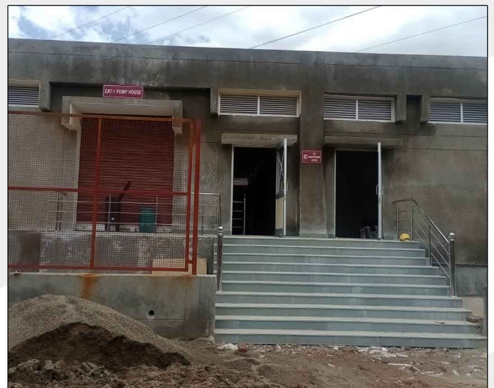
Homogeneous Tank (Pump Room)
