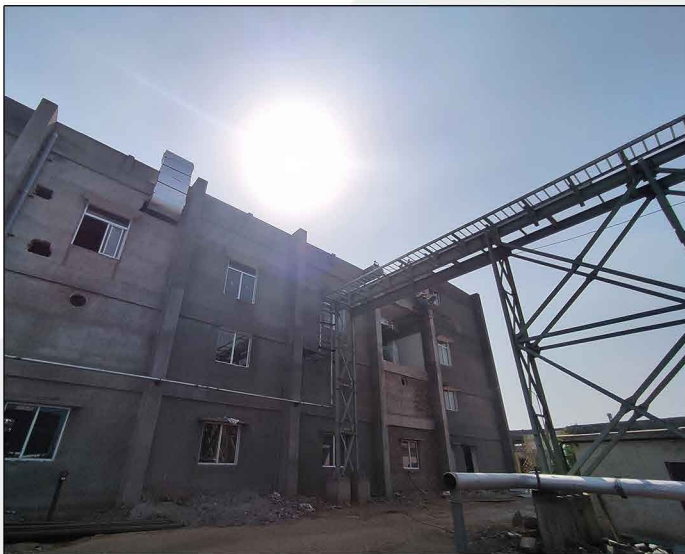
40 TPH Boiler Control Building
