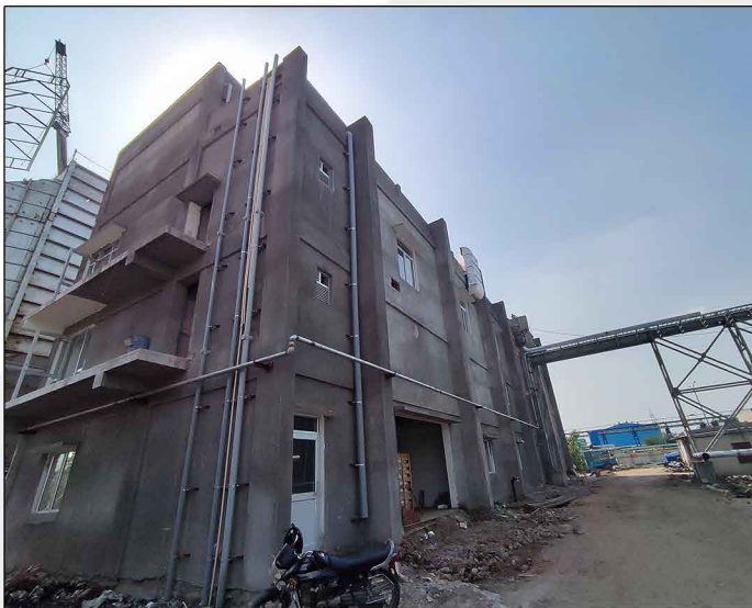
40 TPH Boiler Control Building
