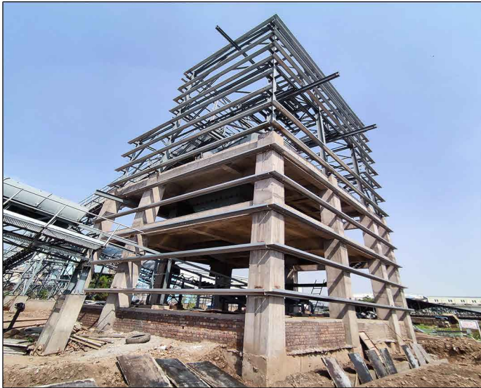
Crusher House & Conveyor (40 TPH Boiler)
