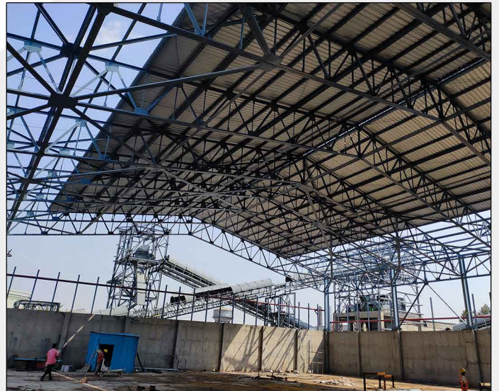
Husk Yard Shed (4000 Sqm)
