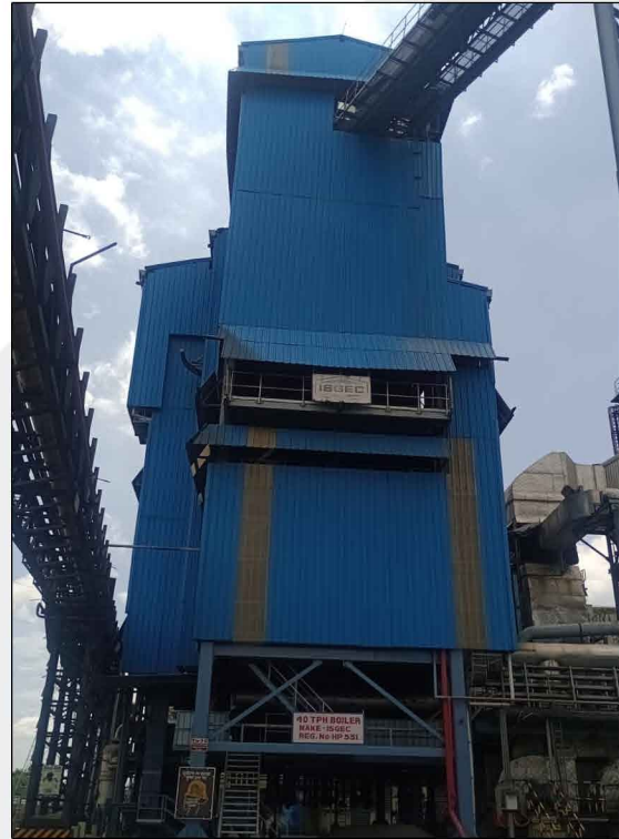
40 TPH Boiler Area
