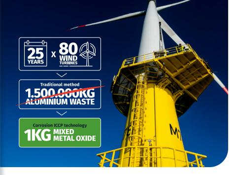
In larger terms, like an entire wind park, the results are even more significant. An average wind turbine park of 80 turbine foundations requires 1,500,000 kg of aluminium anodes versus 0.972 kg of MMO material.
