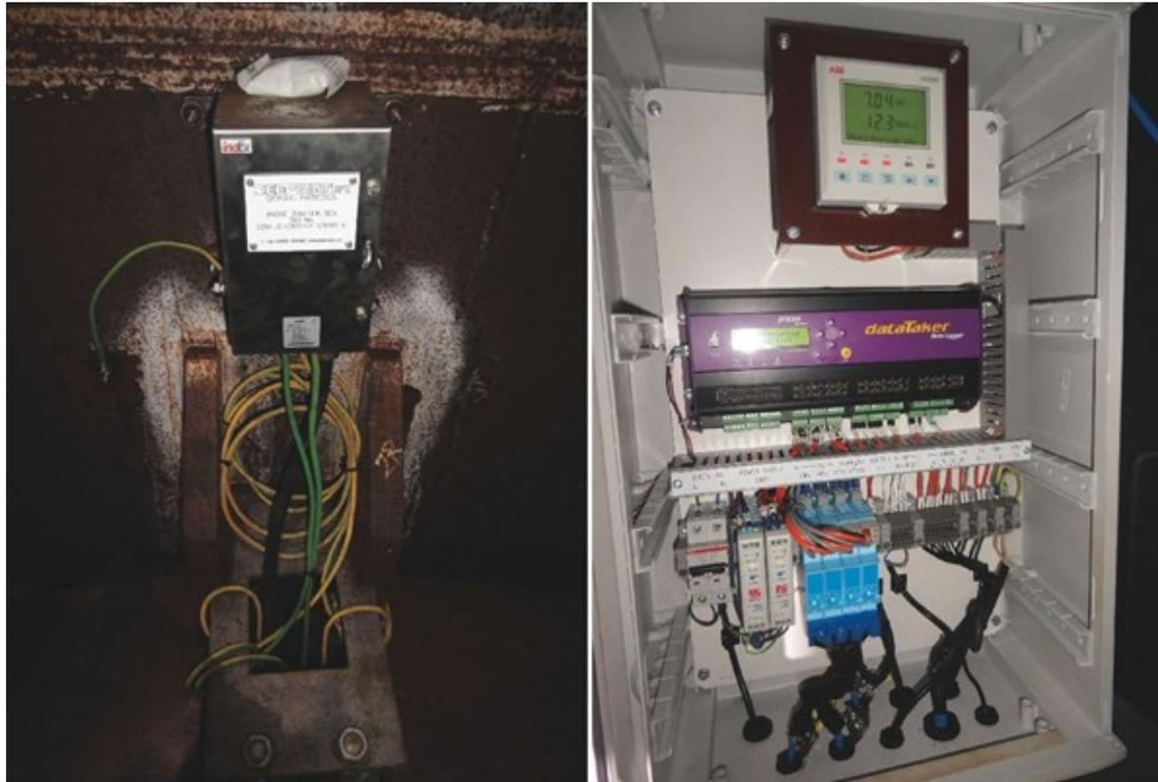
The junction box (left), installed above the lower platform, connects the anodes to the structure. Right, the monitoring system collects data from hydrogen sensors, a CD plate, pH probe, dissolved oxygen probe, and current input monitor to confirm the operation of a ventilation system. Photos courtesy of Alex Delwiche.
