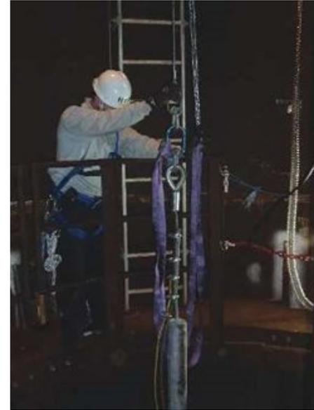
A trial anode string is lowered into the monopile's contained water. Photo courtesy of Alex Delwiche.
