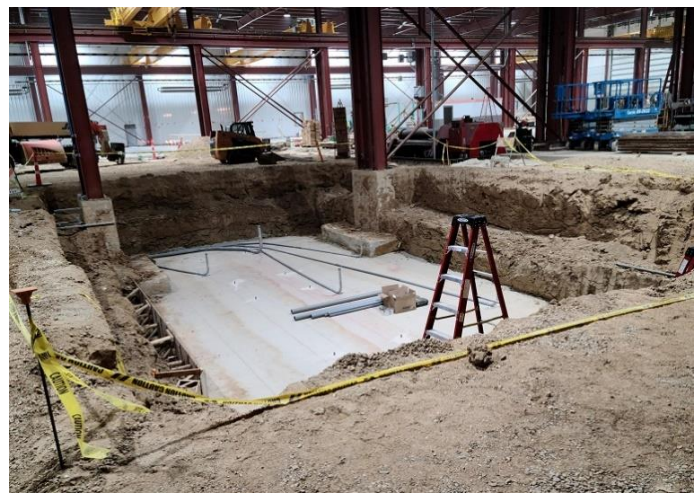
Pit Base & Beginning of Roller Foundation
