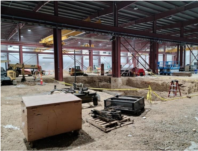
Operation Pit for Plate Roller
