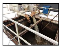
Discharge of Screen Effluent into the Equalization Basin
