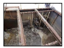
Equalization Basin Showing Pump Rails and Discharge Piping
