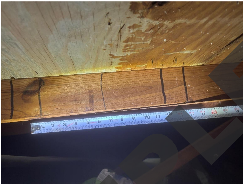
09. Attic (Roof Deck Attachment Spacing @12")
