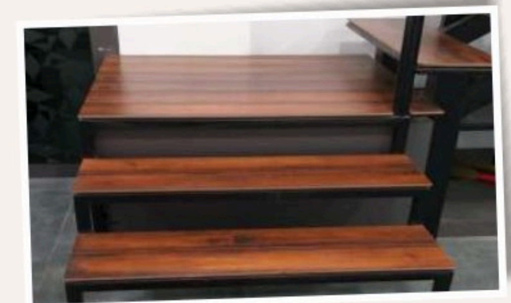
Flooring used in stair case
