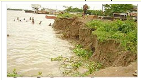
River Erosion due to Flood
