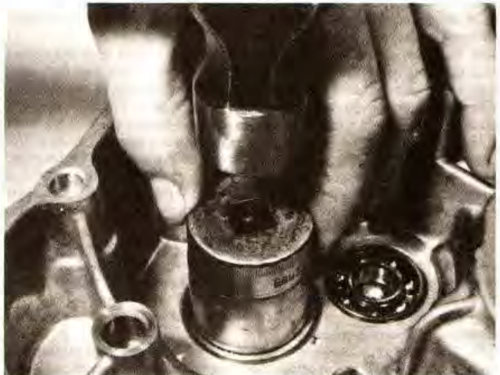
4.92 Using a large socket to drive a new transmission bearing into place
