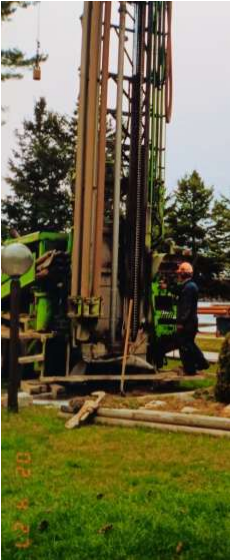
Drilling new well
