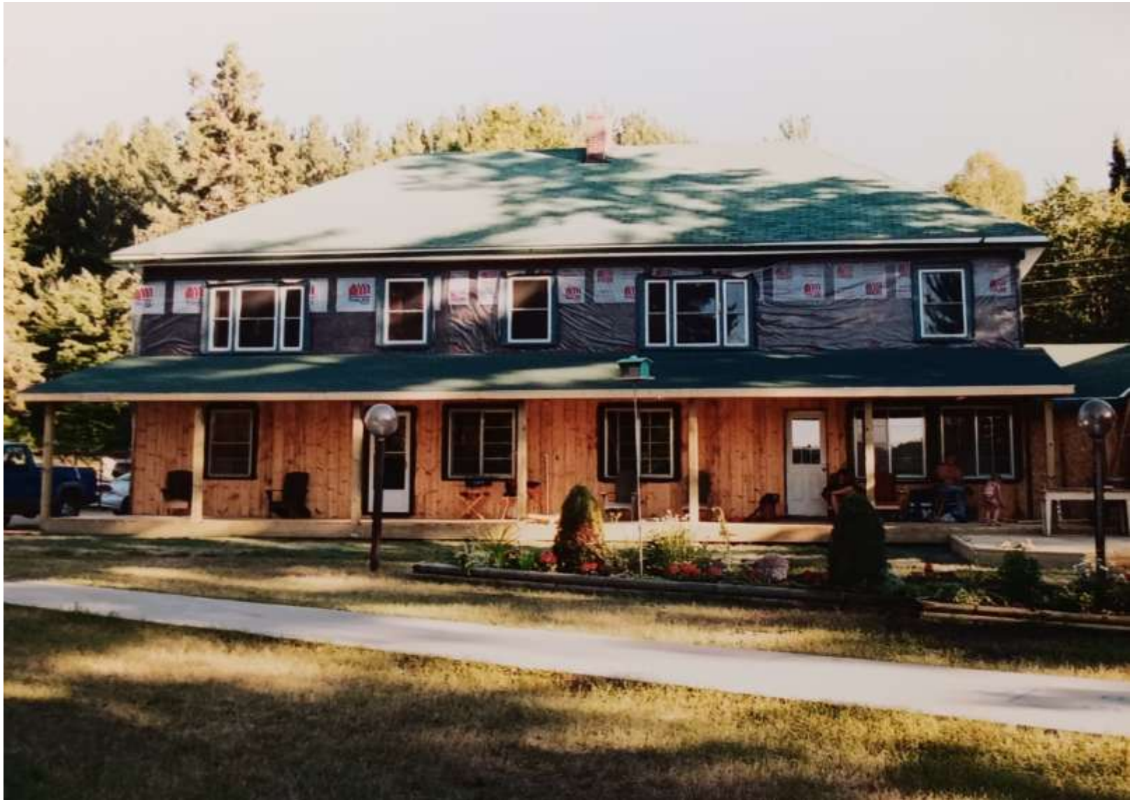
2002 Construction - Main Lodge Photo credit: Brian Middleton
