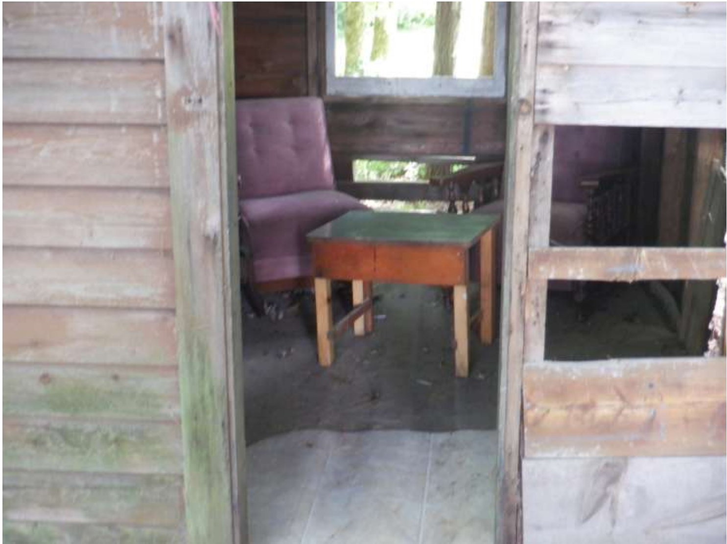
2024 Pump house Photo credit: Paul LaRue
