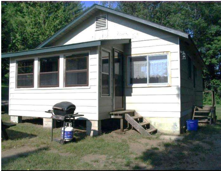
2010 Cedar before deck built
