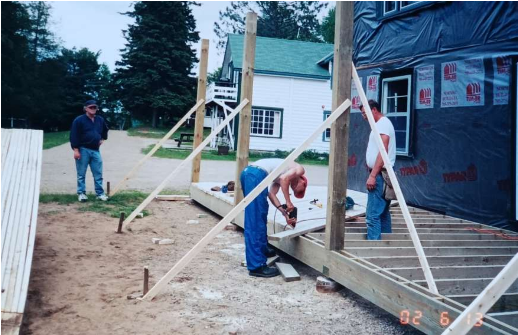
2002 Construction - Main Lodge Photo credit: Brian Middleton
