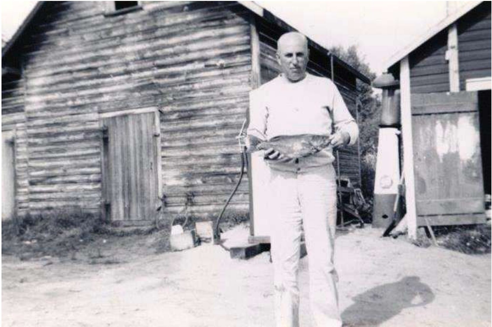
2 nd location of Ice House to the left, Marina storage to the right Photo credit: Bernie Jaroscak
