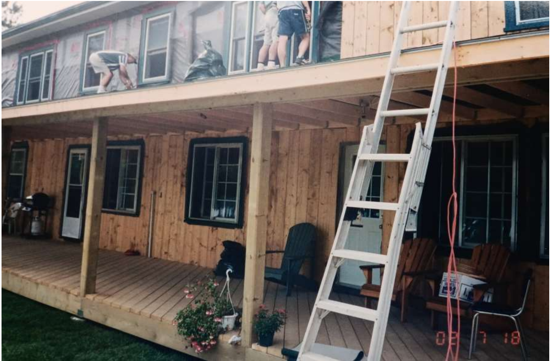
2002 Construction - Main Lodge Photo credit: Brian Middleton
