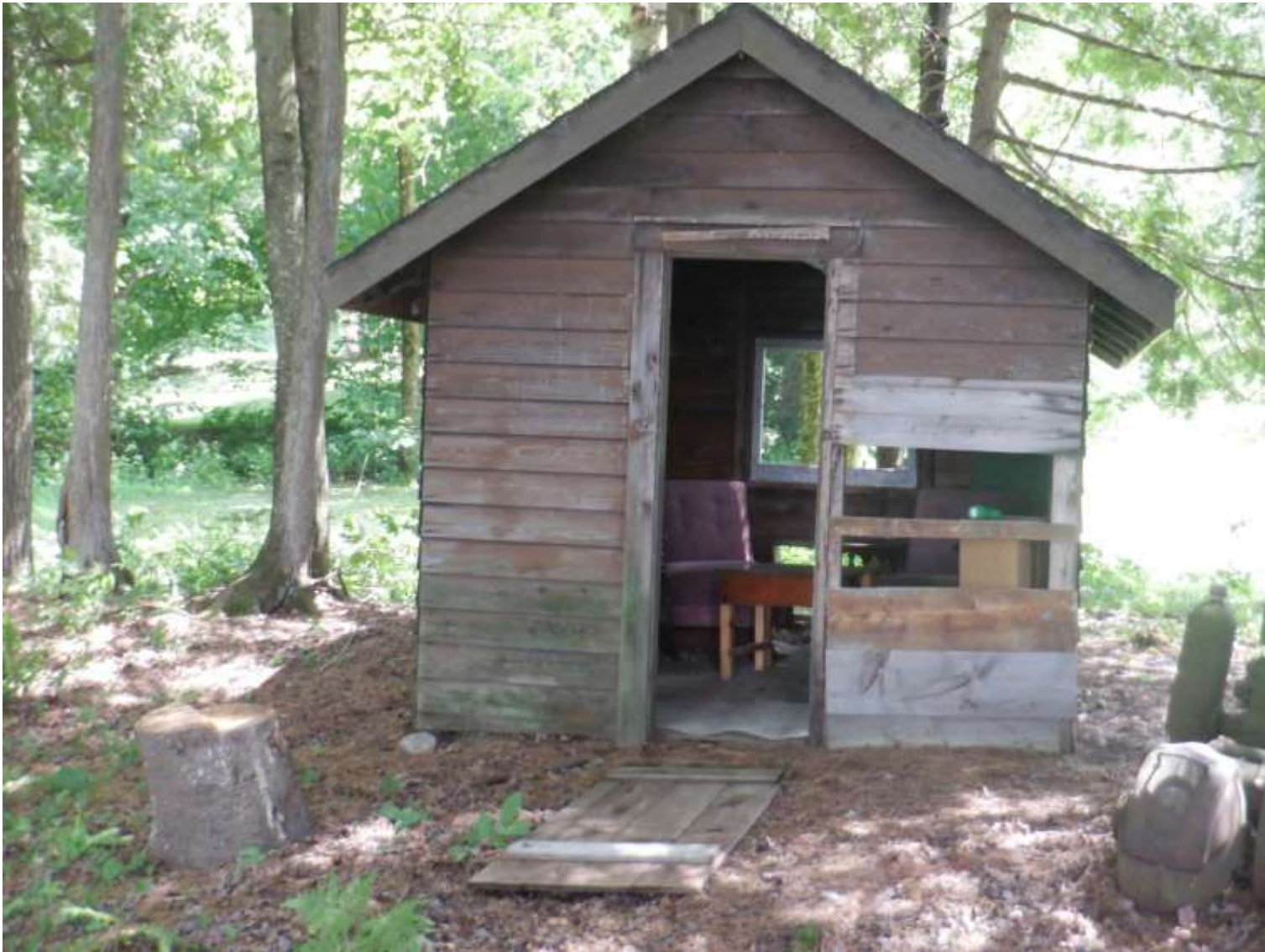
2024 Pump house Photo credit: Paul LaRue
