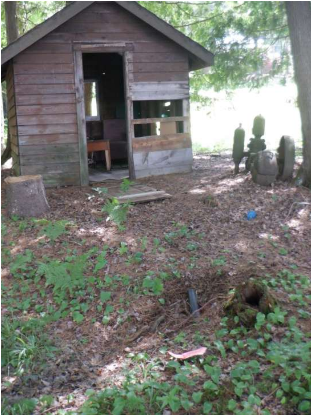
2024 Pump house Photo credit: Paul LaRue
