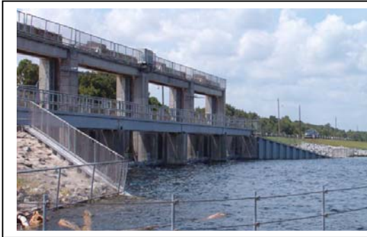
Spillway Structure – Lake Side
