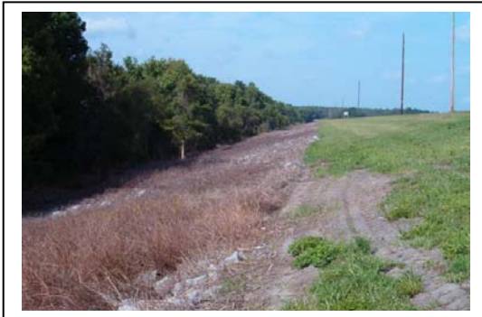
Downstream Embankment Looking Generally West from Spillway
