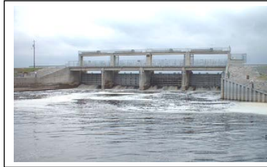
Spillway Structure – Tailwater Side
