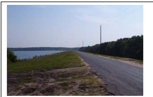
Upstream Embankment Looking Generally East from Near West End of Embankment
