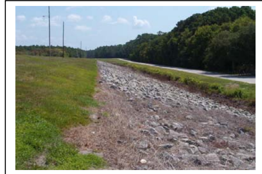
Downstream Embankment Looking Generally East from Near Spillway
