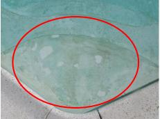
Item 28 •Repair: There is damage at some areas of the decking and coping unions. Recommend sealing and caulking to help prevent water entry.
