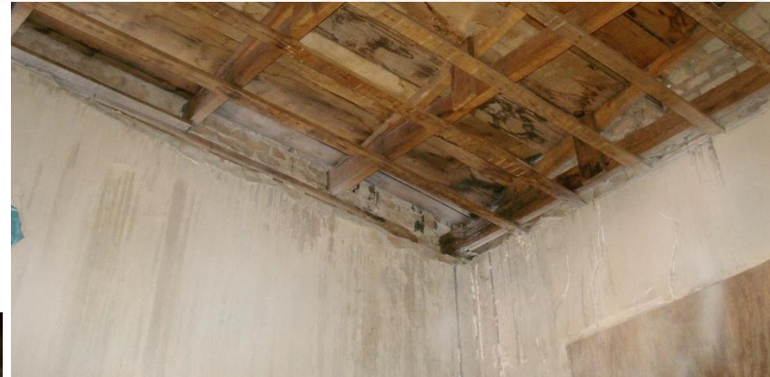
Water damage to walls and ceiling
