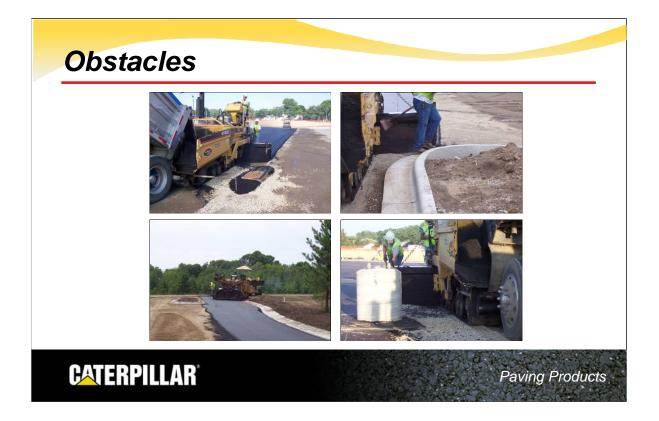
Commercial paving is normally filled with obstacles. Jobs progress most efficiently when planning for obstacles happens at the beginning of a job rather than simply dealing with obstacles as they appear during each pull.
