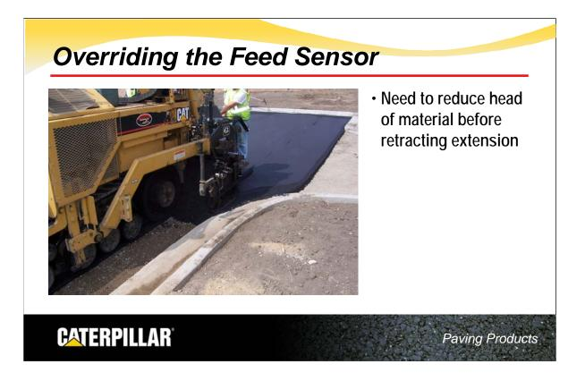
In this view, the screed operator has retracted the left screed extension while paving around an obstacle. Prior to retracting the extension, he overrode the feeder sensor to reduce the head of material. There are two ways to override the feed system.
