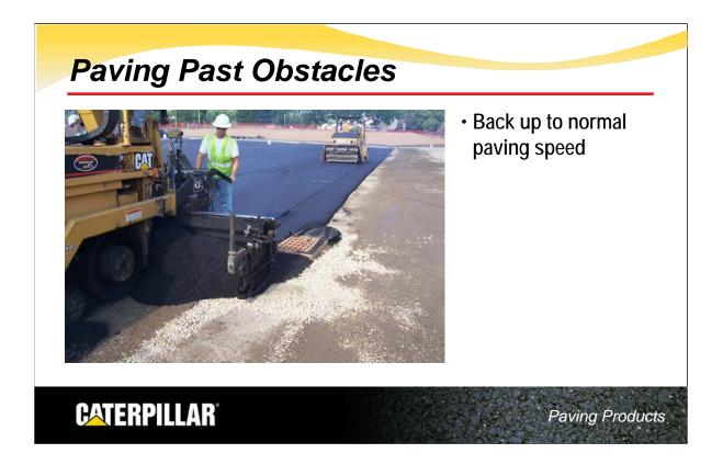
As the paver pulls past the obstacle, the operator normally brings the paving speed back up to the normal range.
