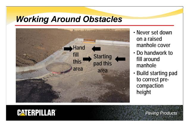
Never set the screed down on a manhole cover. It may look like the right place to start, but a pad built to the correct pre-compaction height is a better choice. Sometimes, no matter how well planned the project, there will be a lot of handwork around obstacles.
