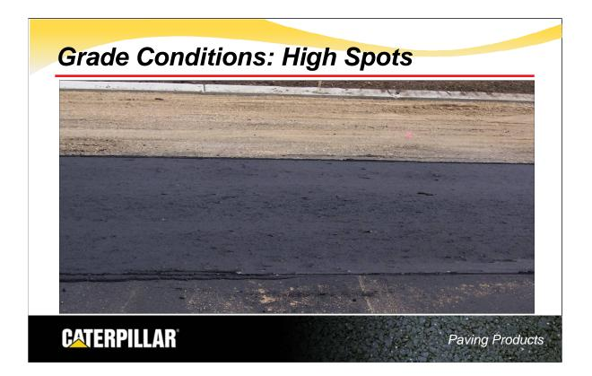
This is a good example of a high spot in the grade. The mat has an open texture with a very poor visual appearance. Compaction will be difficult in this area. Most likely there will be broken aggregates and premature failure. There will probably be a bump in this area so ride comfort will be affected, too. It will be difficult to get full pay for a project with appearance and quality issues like this.
