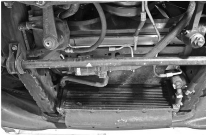
Photo showing steps 25 and 26 completed.
