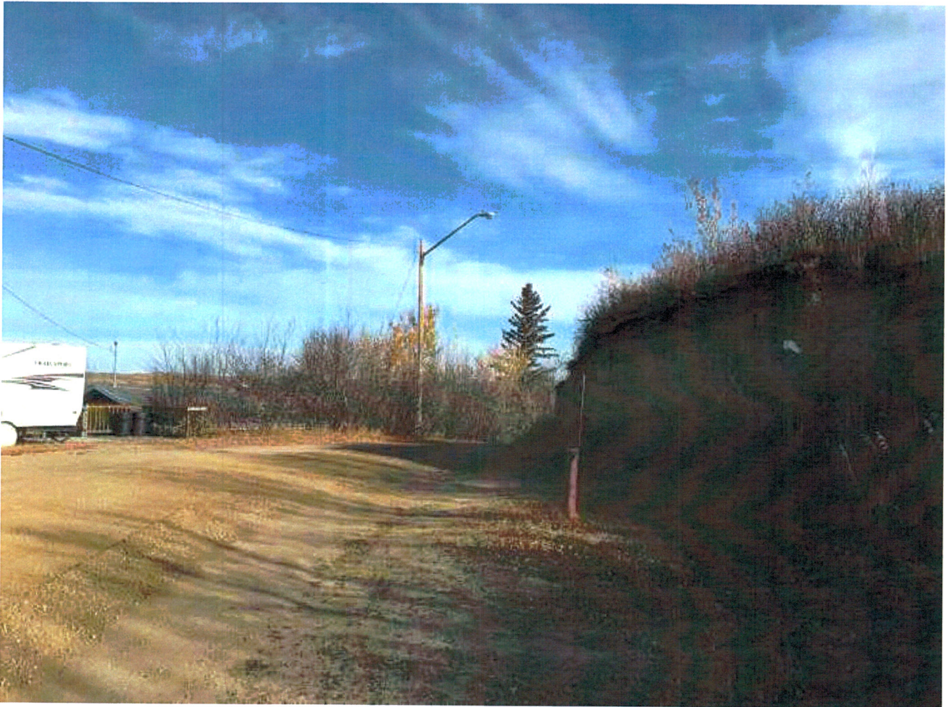
Figure 5: Exposed cliff, north end of Archdekin Drive, silty sand with some clay.
