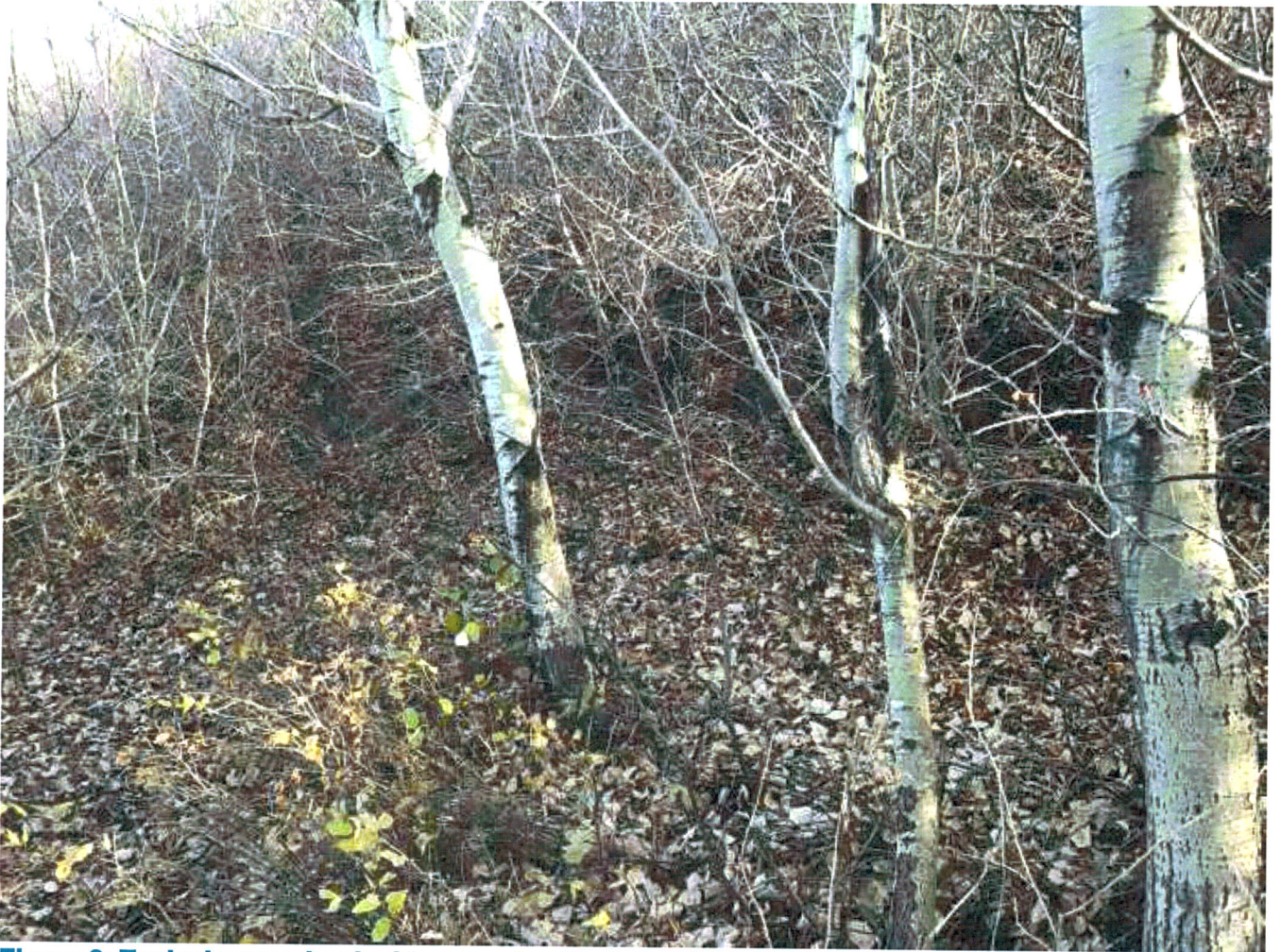
Figure 2: Typical scarp, hooked tree trunks. Upslope of the north end of Archdekin Drive.
