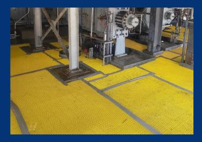
Specs: 200 mil thickness 3/8" small diamond pattern prevents material, debris and tool falls
