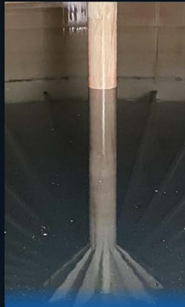
Tank & Reservoir Inspections
