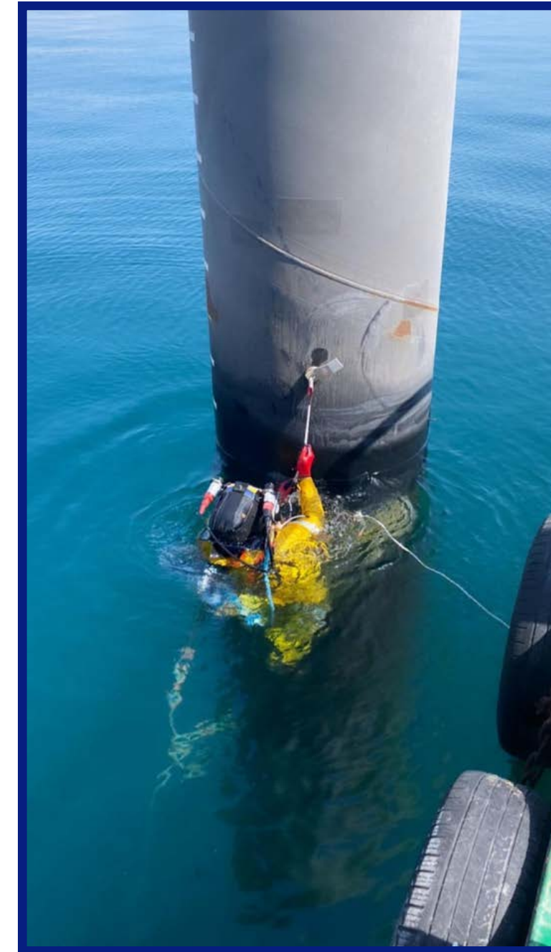
ANODE INSTALLATION ON A PILE
