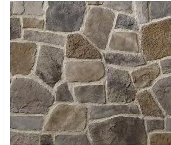
PALISADES ANCIENT VILLA LEDGESTONE 1/2" mortar joints
