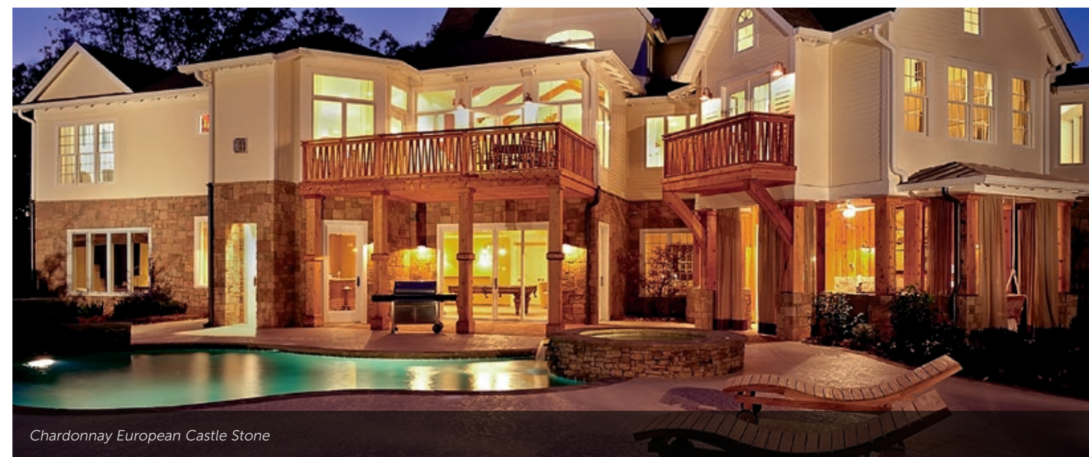
Chardonnay European Castle Stone tight-fitted mortar joints
