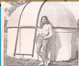
BACKYARD OBSERVATORY - Lisa Schneider, a granddaughter of Mr. Goetz, stands beside her grandfather's backyard observatory from which the moon shot with its controversial "object" was taken. The structure, 8 feet in diameter and 6 feet in height, was constructed by Mr. Goetz using hardware and plywood. The hand-operated turn with the center sliding panel revolves at a 360 degree.
