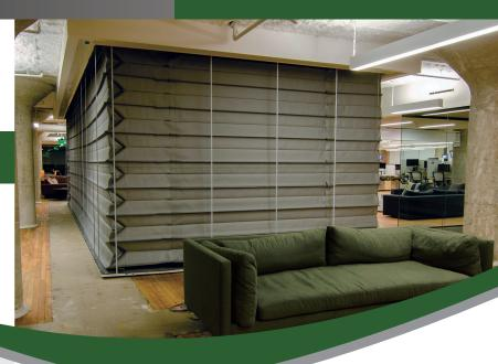
Codes and Standards. M4000 fulfills IBC requirements to provide an opening protective, where these assemblies are permitted as passive barriers used smoke control systems. This fire-rated curtain system can serve as opening protective certain applications in atrium, stairwell and escalator construction.
