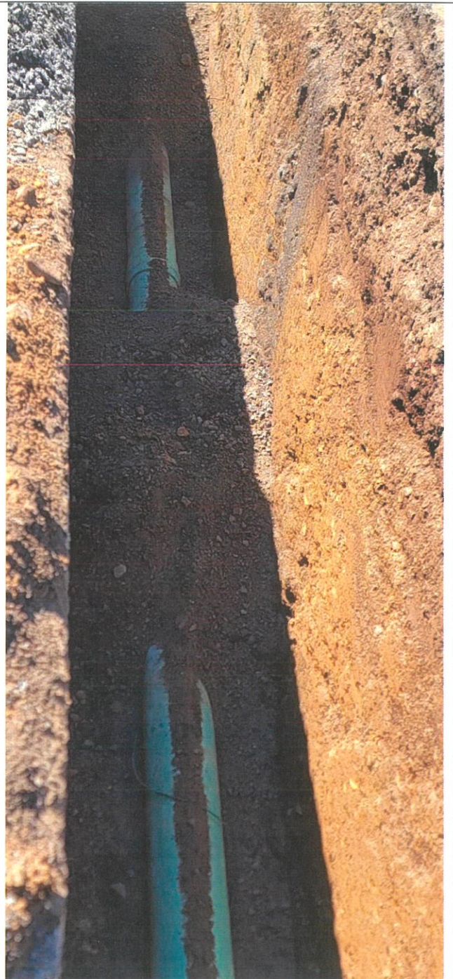
Backfill in sewer trench, May 18, 2026
