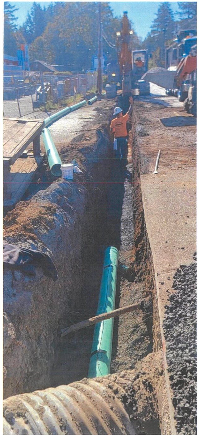
Laying sewer pipe on Caves Highway, May 18, 2026
