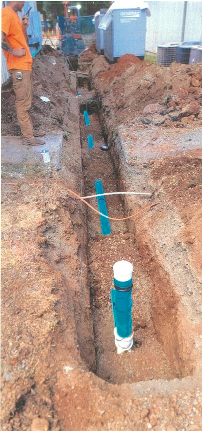
Installing water and sewer infrastructure on IVFD property between the two buildings, May 14, 2026
