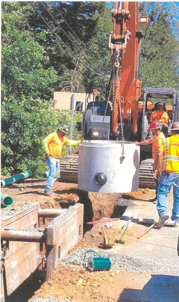
Installing one of three sewer manholes on Caves Highway, May 18, 2026
