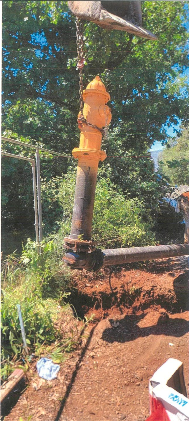
Installing one of three hydrants on Caves Highway, this one in front of the fire station, May 7, 2026
