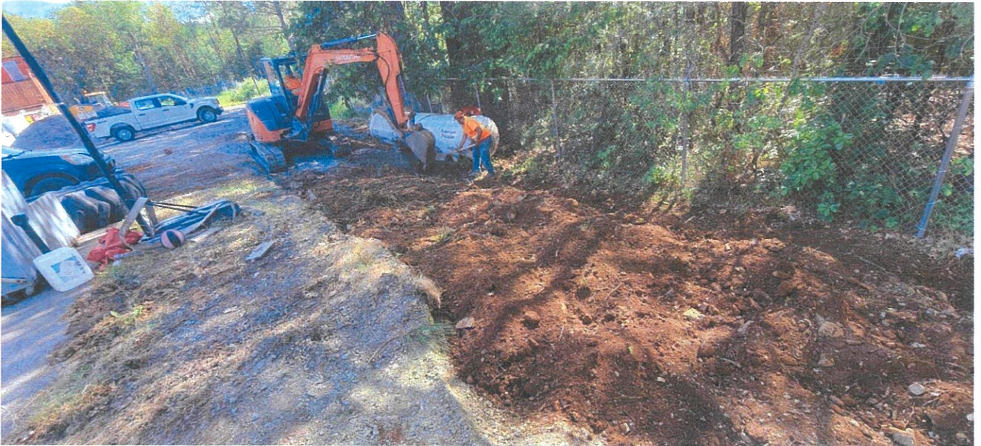
Trenching water line on west side of IVFD property, May 13, 2026
