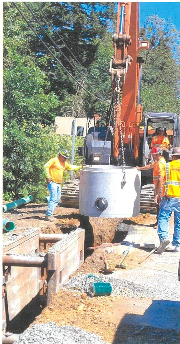
Installing one of three sewer manholes on Caves Highway, May 18, 2026
