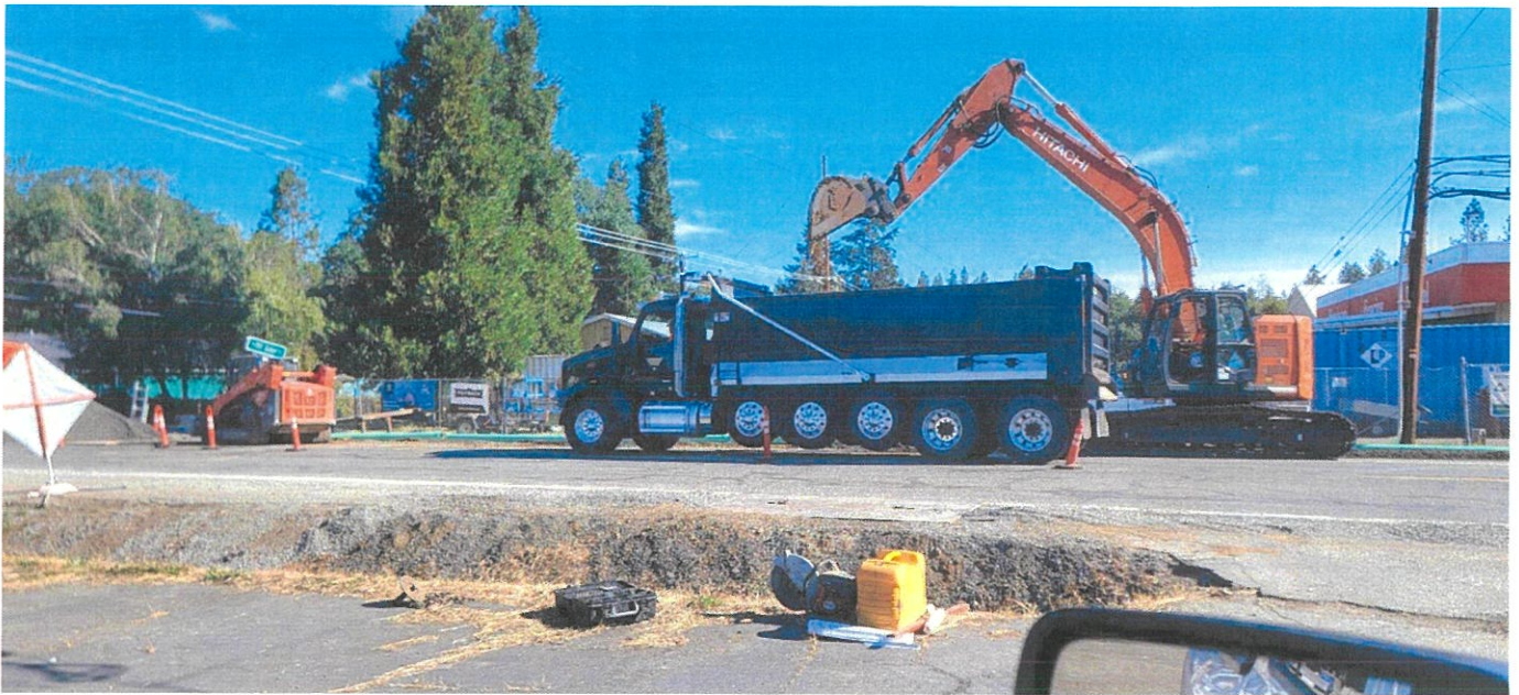
Work on sewer line on Caves Highway, May 18, 2026
