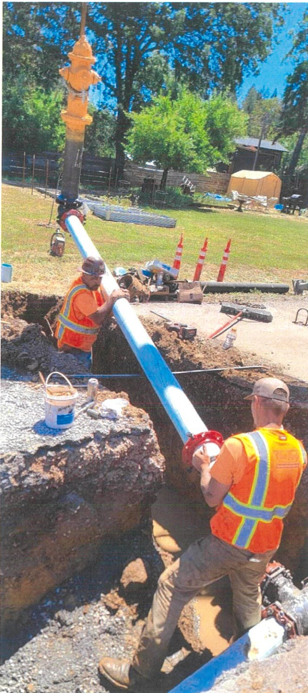
Installing one of the three hydrants with the water line on Caves Highway, May 21, 2026
