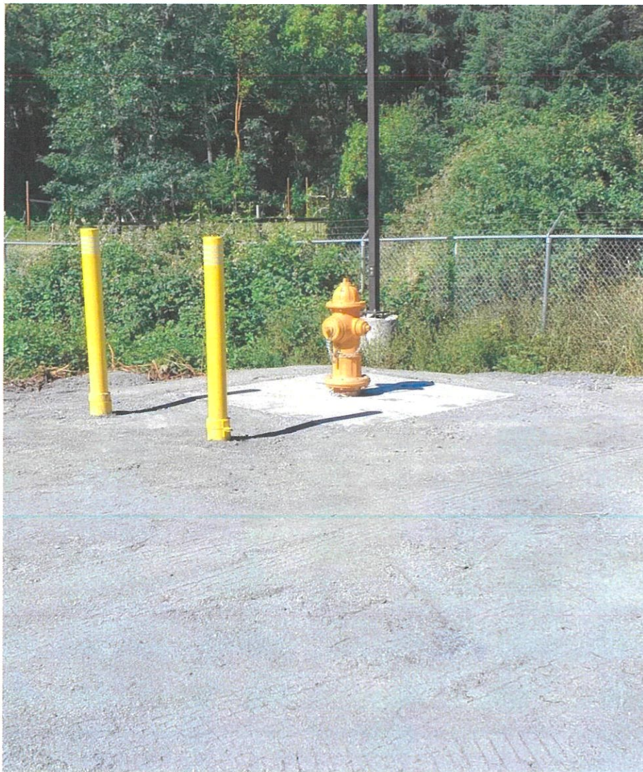
Finished hydrant and bollards on concrete pad in IVFD training area, May 28, 2026
