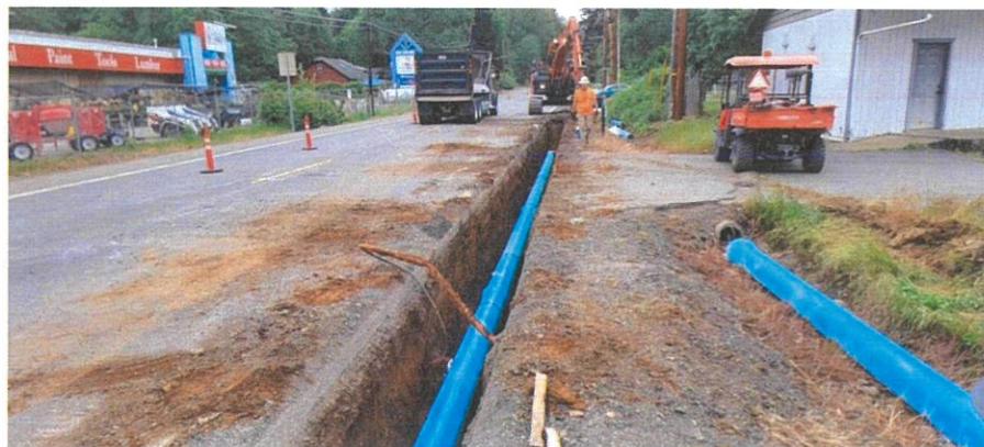
Laying water pipe, May 5, 2026
