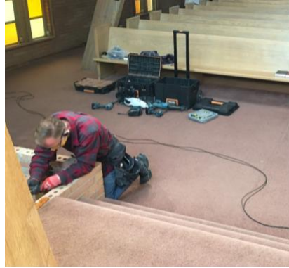
Burke Jackson installs wiring under the Chancel
