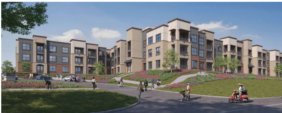
Palladium USA is underway on construction of Embree Eastside, a 107-unit mixed-income development in the northeastern Dallas suburb of Garland. The project team includes the Garland Housing Finance Corp. Units will be reserved for households earning between 30 to 60 percent of the area median income. PNC Bank provided equity and construction financing.
