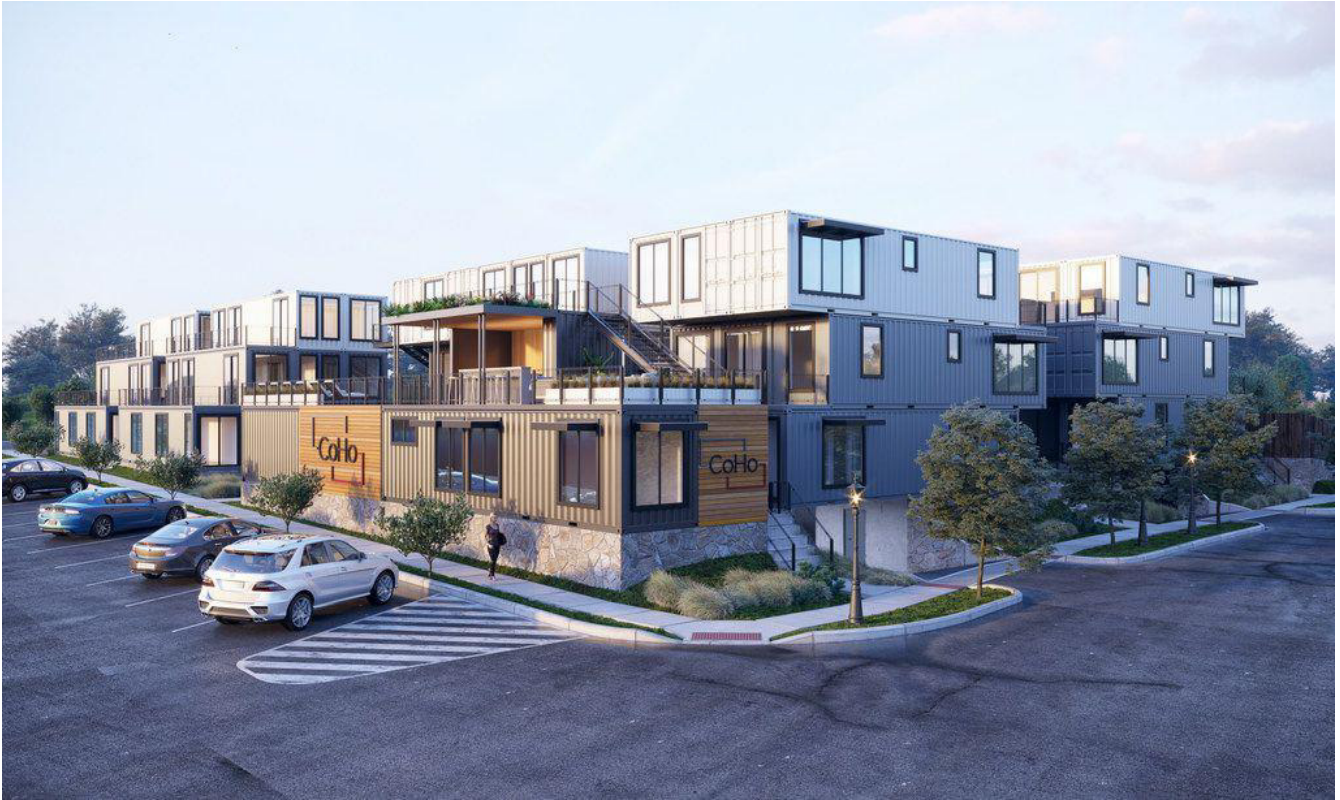
A 34-unit apartment project south of downtown Fort Worth is being constructed out of 76 steel shipping containers. (Keywinn Development)
