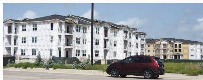
Apartments in progress stand on Palladium USA property on Friday, July 23. The four apartment buildings planned will have 183 units total, most of which are designed for workers of modest means, according to senior vice president and COO Fred D'Lizarraga. The first building is planned to be completed by the end of the year. Staff Photo by Graysen Golter
