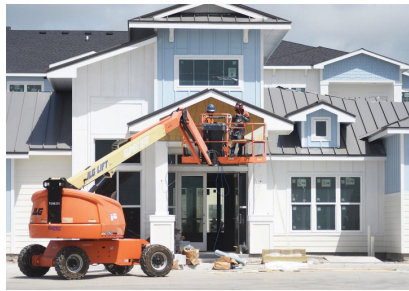
Construction workers continue work on a building within the Palladium Apartments property on Friday, July 23. Staff Photo by Graysen Golter
