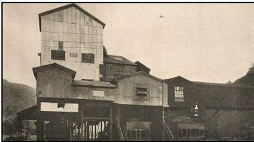
The tipple at the MacAlpin Mine (used to load extracted coal for transport into railroad hopper)
