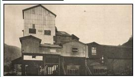
The tipple at the MacAlpin Mine (used to load extracted coal for transport into railroad hopper)
