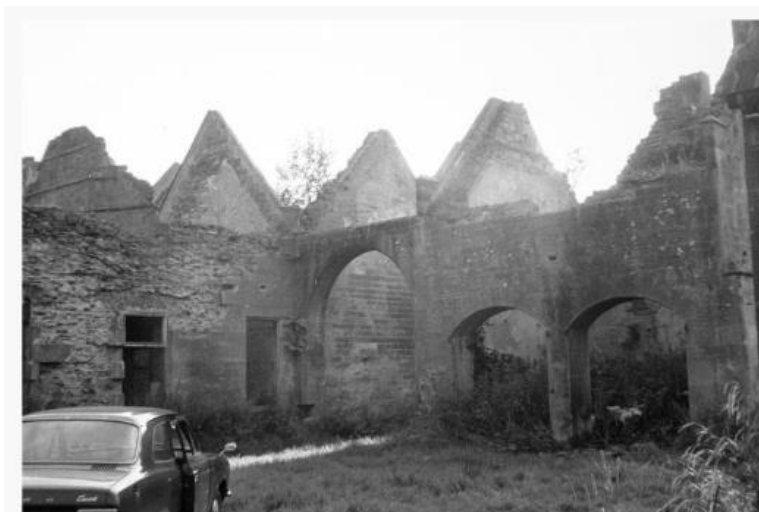
Poltalloch House, General view of house in gutted state
