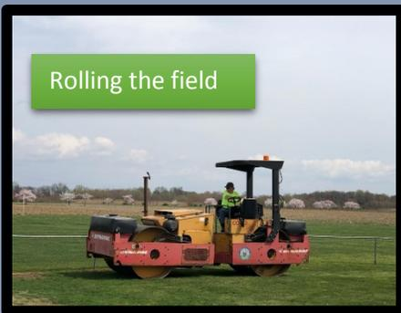
*The County rolled the runway & surrounding field areas and filled in low spots with fresh top soil and seeded. The dip in the middle of the runway that runs across the field was filled in. That should really help our planes complete a smooth landing and rollout to a full stop.*
