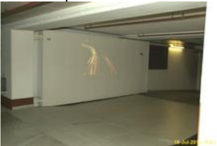
Large fire door, sealing a fallout and air raid shelter inside the basement parking garage of a hotel in Germany.
