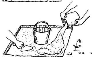
6. Remove the bucket when the cement is beginning to get hard (about 3 hours). Then cover the cement with damp cloths, sand, hay, or a sheet of plastic and keep it wet. Remove slab after 3 days.
