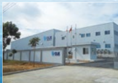
Cold Storage Warehouse in Vietnam
