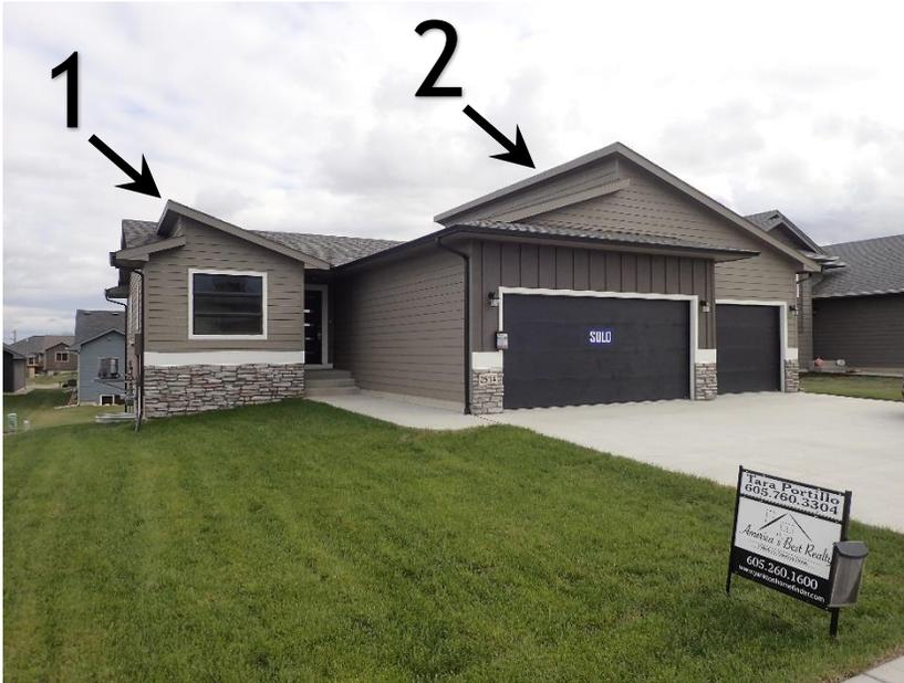
Apex 1 has a standard drip edge installed which is unacceptable for this type of installation.
