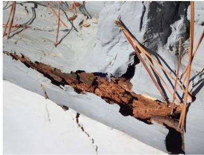
Rotted window frames. The photo on the left is the north window in the upstairs hallway. This window is covered with caulking to prevent leaking through the rotted areas.
