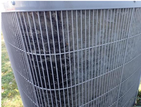
The coils on the heat pump need cleaning.
