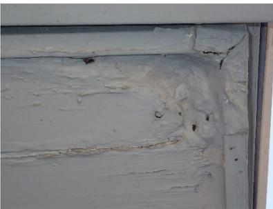
This is the underside of the soffit on the northeast corner of the structure. The soffit has been filled with caulking and the soffit and fascia are rotten.
