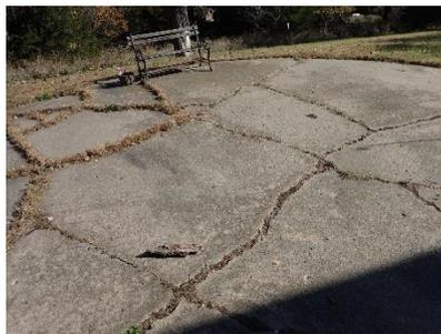
The sidewalks, patio and driveway have excessive cracking and there are areas of the patio that slope to the foundation.
