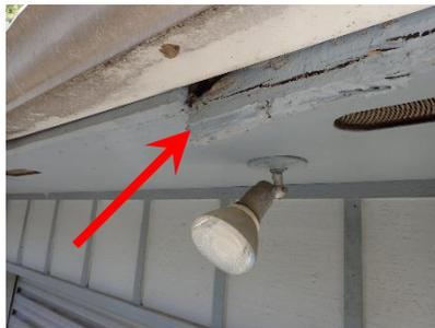
Damaged gutter and fascia above garage door.
