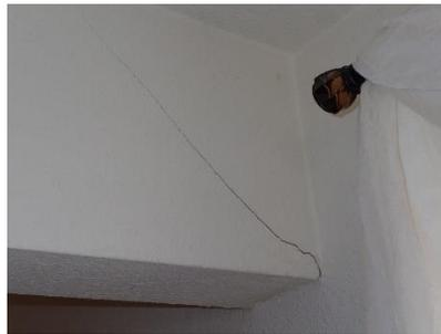
Significant settlement cracks were observed around the beam supporting the floor joists above.
