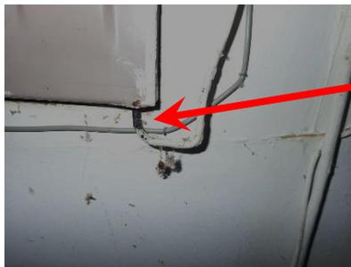
This wire is entering the panel between the cover and the panel body. If the insulation becomes damaged the panel can become electrified and be a shock hazard.
