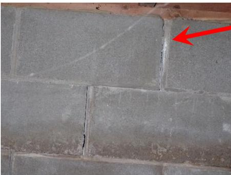
There is a significant step crack on the east wall of the crawlspace. The crack is large enough to see daylight in the areas above grade.
