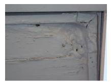
This is the underside of the soffit on the northeast corner of the structure. The soffit has been filled with caulking and the soffit and fascia are rotten.
