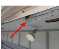
Damaged gutter and fascia above garage door.
