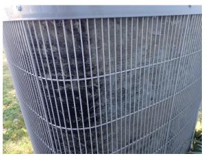
The coils on the heat pump need cleaning.
