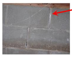
There is a significant step crack on the east wall of the crawlspace. The crack is large enough to see daylight in the areas above grade.
