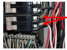
The white and black wires are rated for 20-amps and this is a 40amp breaker. An electrician needs to repair this defect.
