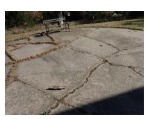
The sidewalks, patio and driveway have excessive cracking and there are areas of the patio that slope to the foundation.
