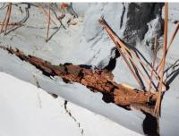
Rotted window frames. The photo on the left is the north window in the upstairs hallway. This window is covered with caulking to prevent leaking through the rotted areas.
