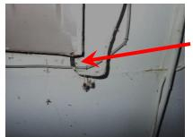
This wire is entering the panel between the cover and the panel body. If the insulation becomes damaged the panel can become electrified and be a shock hazard.
