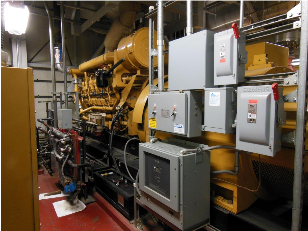
UW Seattle Campus 2 MW Diesel Generator
