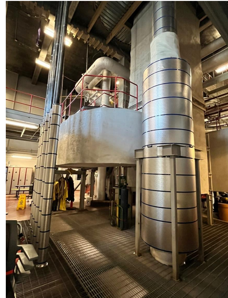
DRUPS coolant lines and exhaust silencer.
