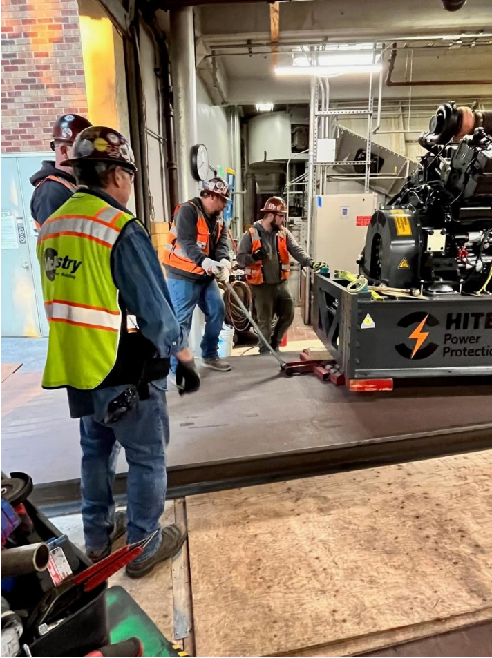
DRUPS diesel engine skid rolled into position.
