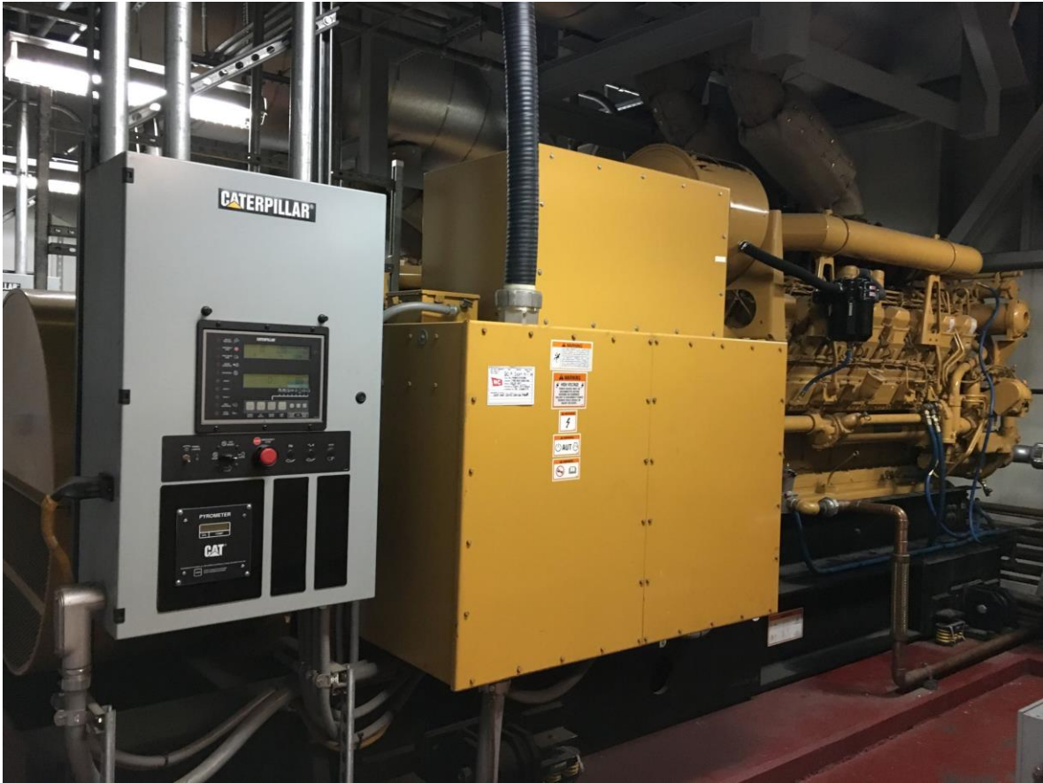
UW Seattle Campus 2 MW Diesel Generator
