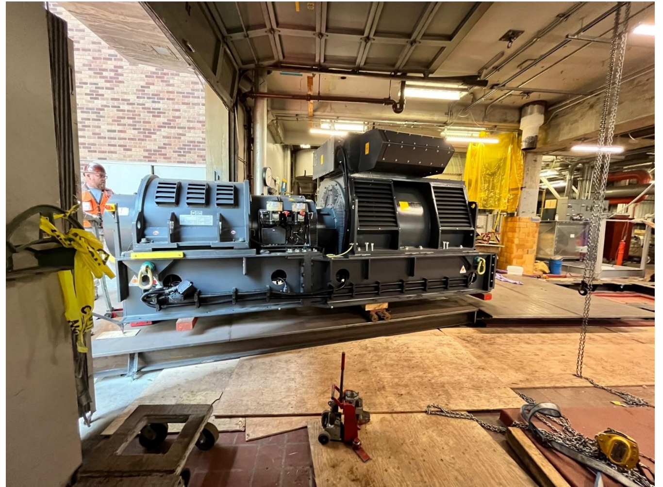
The 20 ton DRUPS generator and Kinetic Energy Module skid rolled into position.
