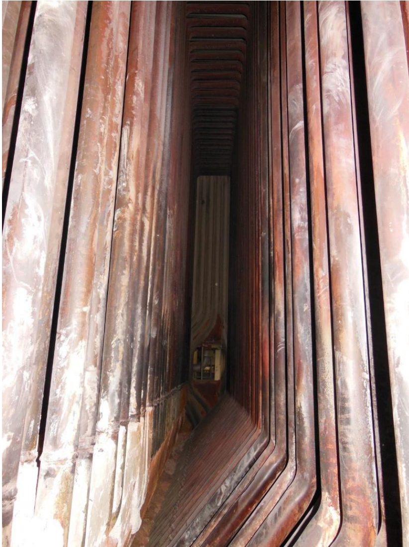
Superheater Removal Before and After
