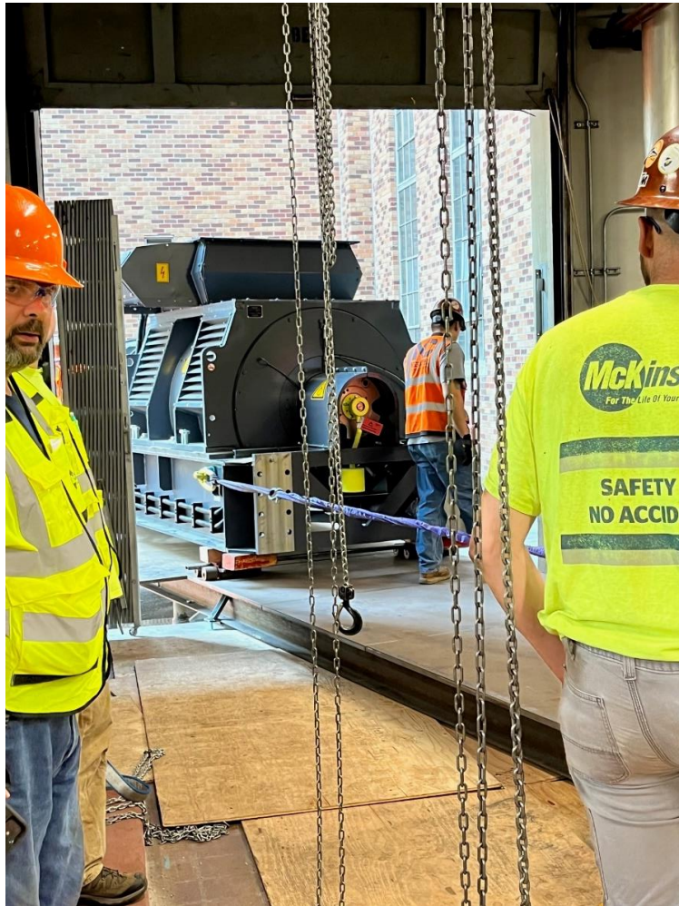
The 20 ton DRUPS generator and Kinetic Energy Module skid rolled into position.
