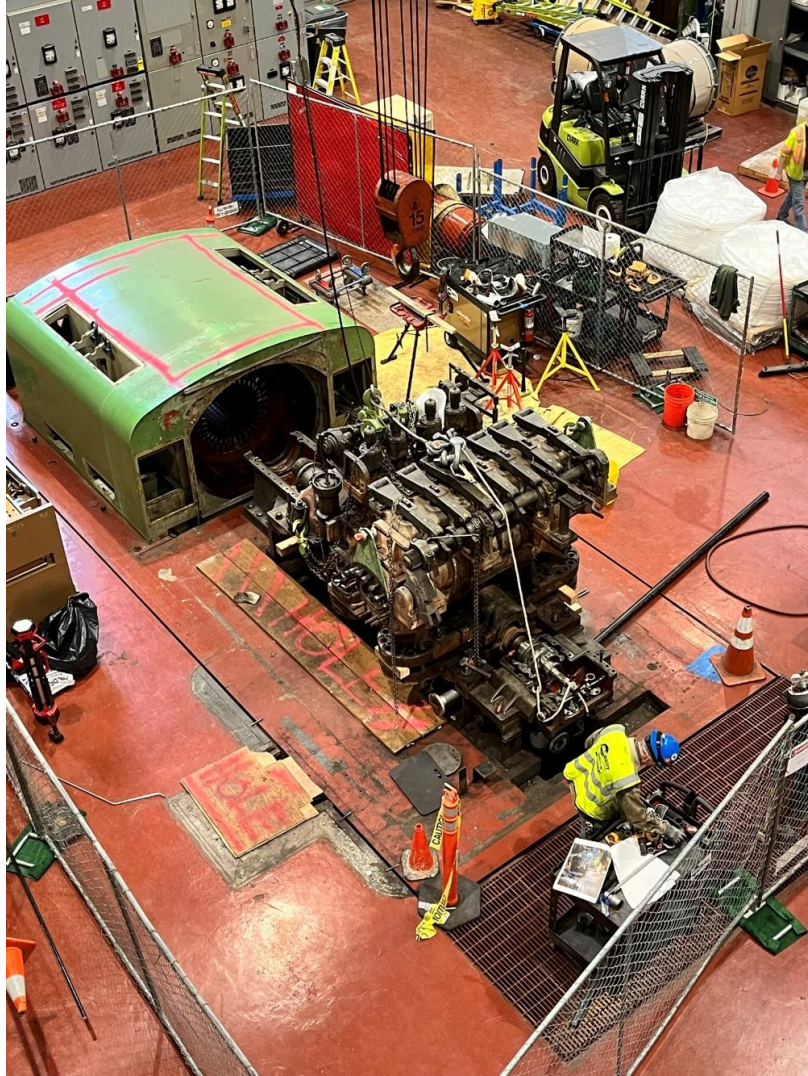
Removal of the upper half of the turbine case.
