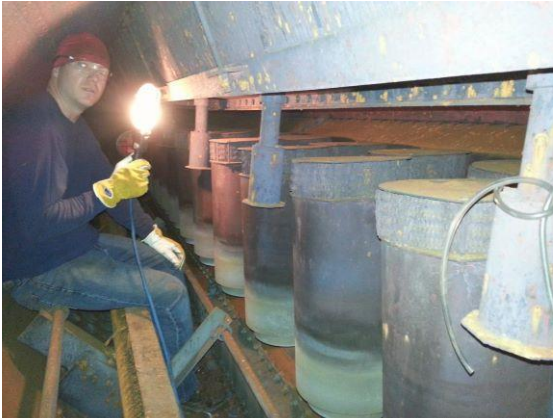
Steam drum before and after modification
