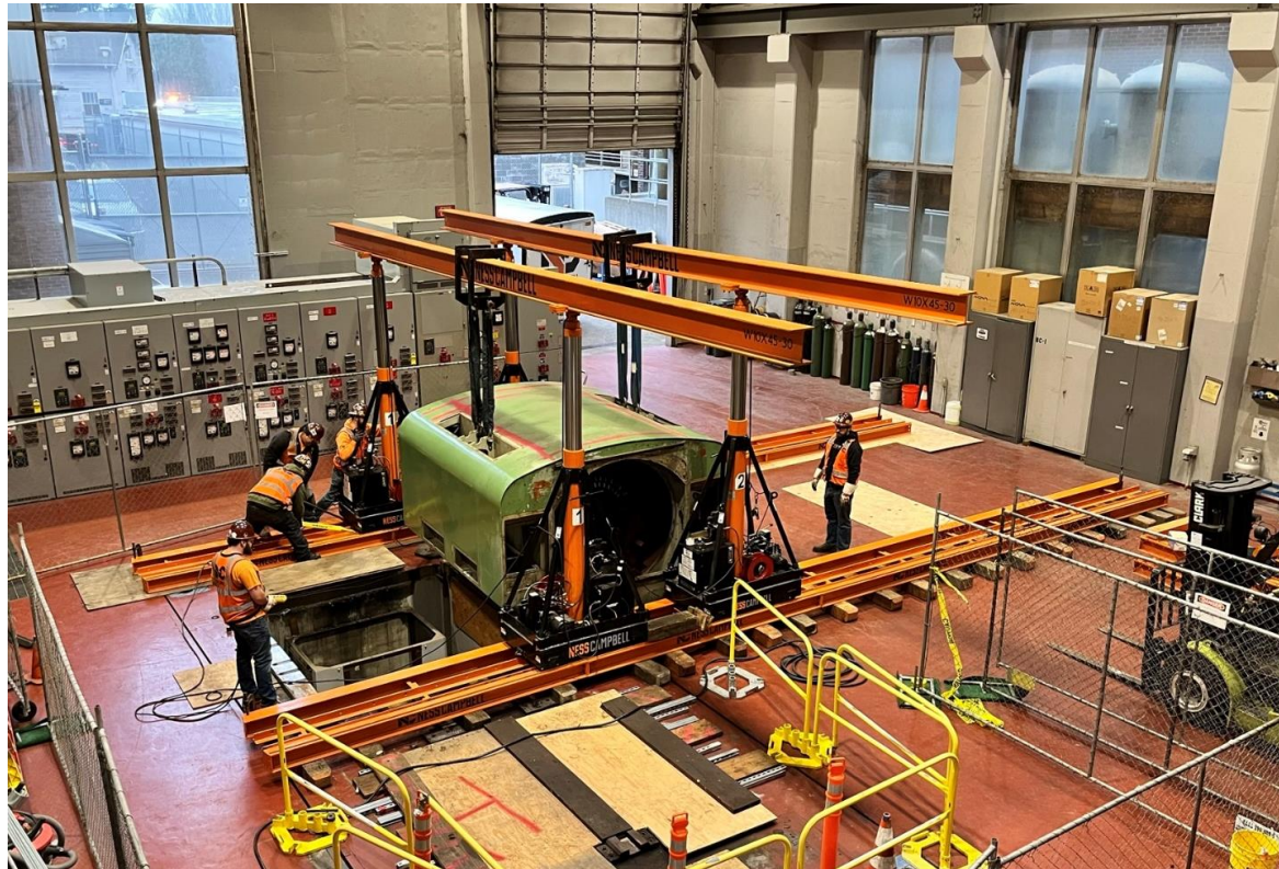
Removal of the 15 ton generator Stator assembly
