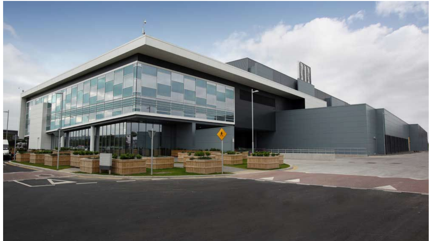
Microsoft Dublin Datacenter
