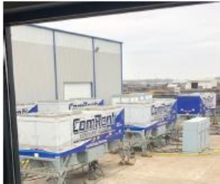
Turbine Test 30MW at 13.8kV
