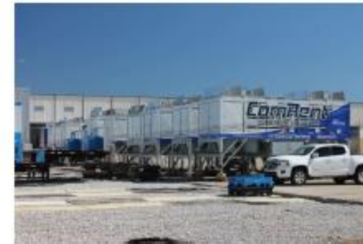
Turbine Test – GE LM6000 50MW at 11kV
