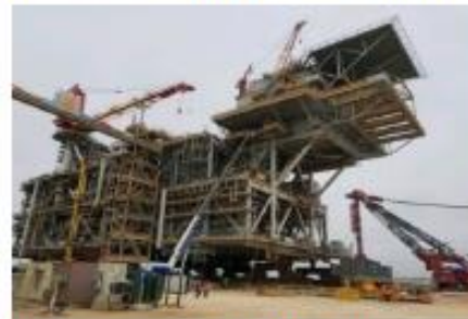
Turbine Test – (3) 7.4 MW Solar Turbine 8.8MW/11MVA at .8pF 50hz at 6.6kV
