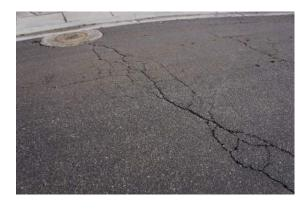
This component provides funding to crack seal and slurry seal. Asphalt is cracking badly in some spots and needs to be done soon.
