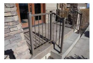
With proper maintenance these railings should last a long time, however these appear to have never been painted or maintained. Fair to poor condition.
