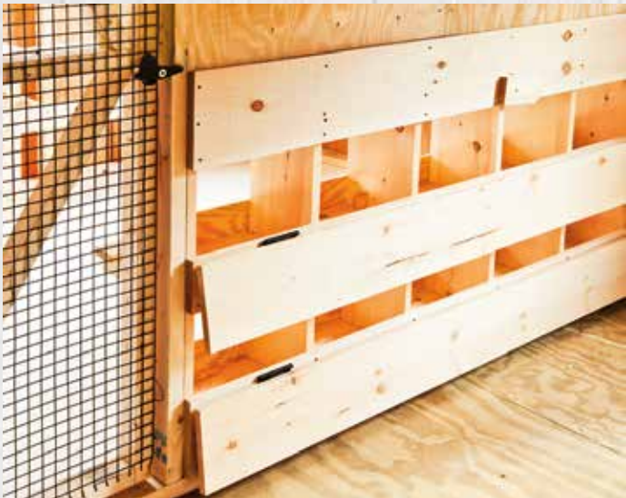
Feed room view of A60 & A80 (pages 38-39)
