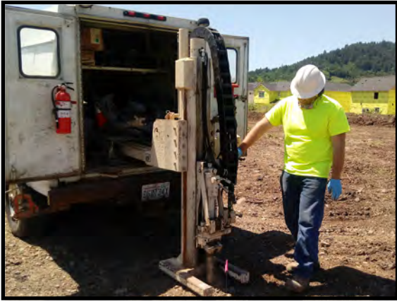
Looking southeast; advancing Soil Boring SG5 by direct push.
