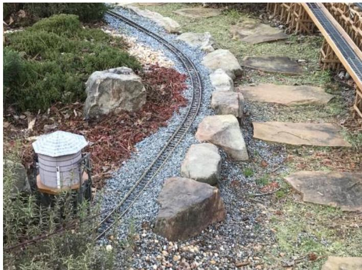
Another outdoor project. Physical upgrades in several places that experience washouts. I have a couple areas that are raised from grade level. The ballast slides down the side and the track goes out of level. I've been building retaining walls that hold the ballast at track level. - Russ Bundy
