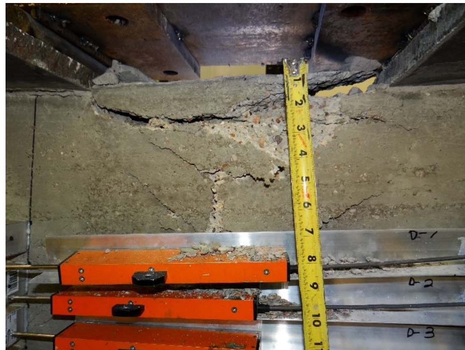
RC #1 beam (Grade 60 steel)
