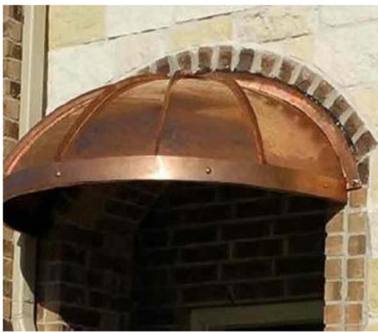
Example of Copper Canopy (Construction)
