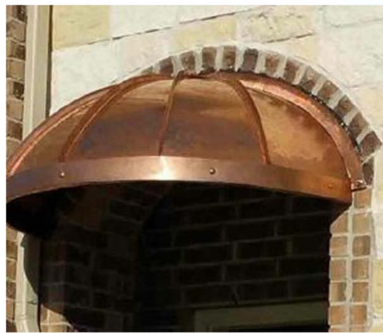
Example of Copper Canopy (Construction)
