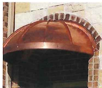
Example of Copper Canopy (Construction)
