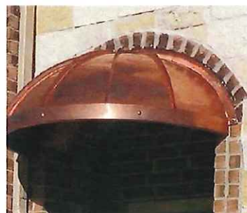
Example of Copper Canopy (Construction)
