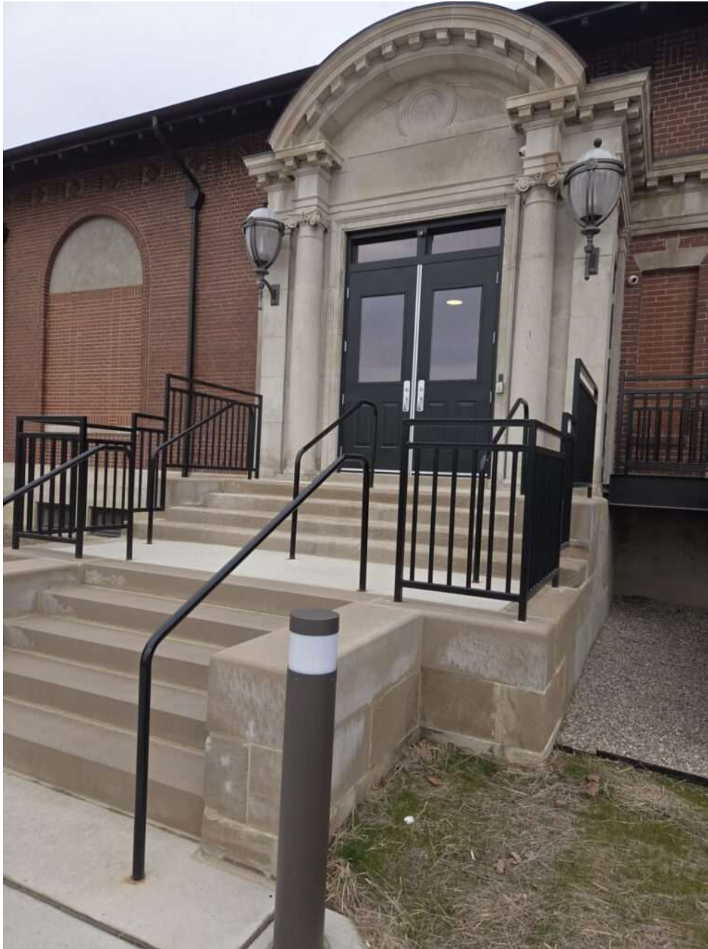
The entrance to KRONK Gym at the Brewster-Wheeler Recreation Center
